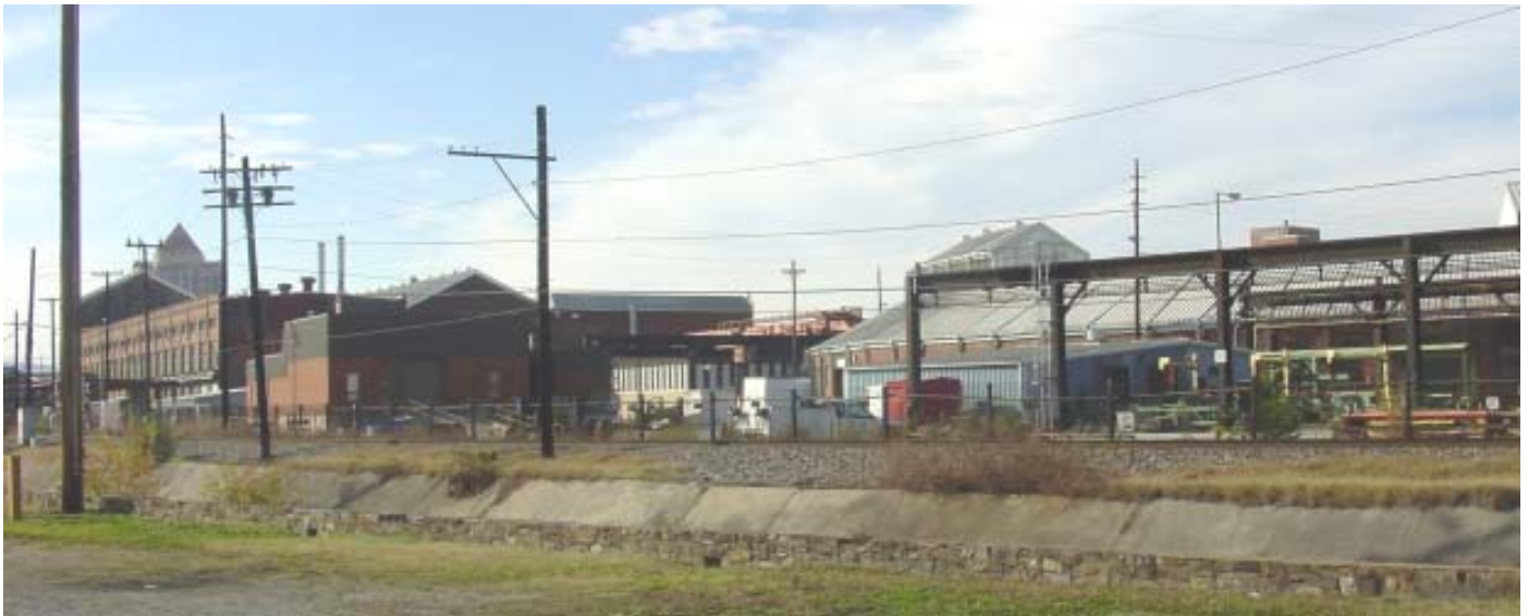
Much of the industrial development in the neighborhood occurred near the Norfolk & Western shops.
