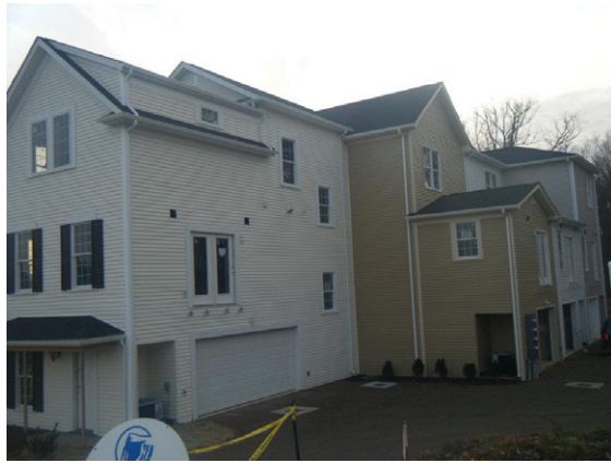
Back-of-house activity zone, Colonial Green, Roanoke, Virginia
