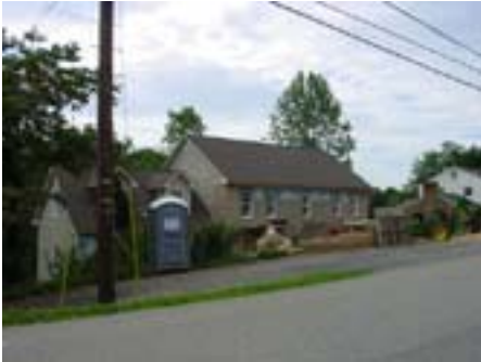
New Construction on Winding Way Road
