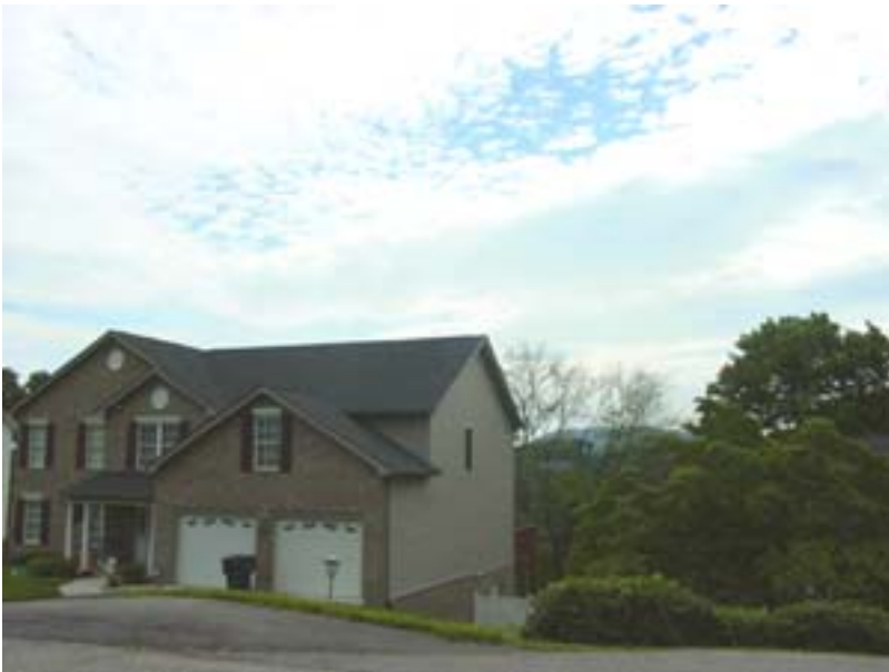
House on Winding Way Road
