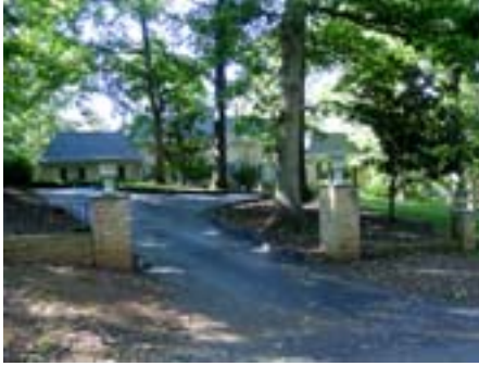
House on Winding Way Road
