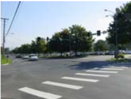
Recently repaved Colonial Avenue near Virginia Western
