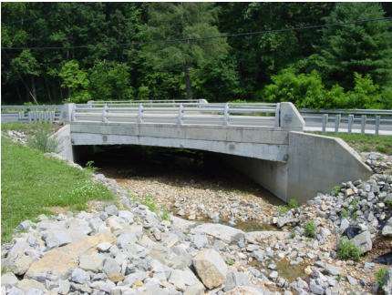
Bridge over Gum Spring Branch
