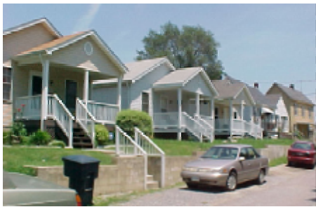
Homes on Staunton Avenue, in the Washington Park neighborhood.
