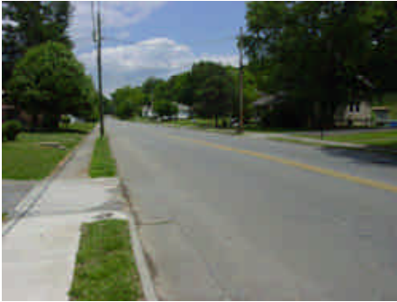
King Street has curb, gutter and sidewalk on its western end, but is still a rural collector street
