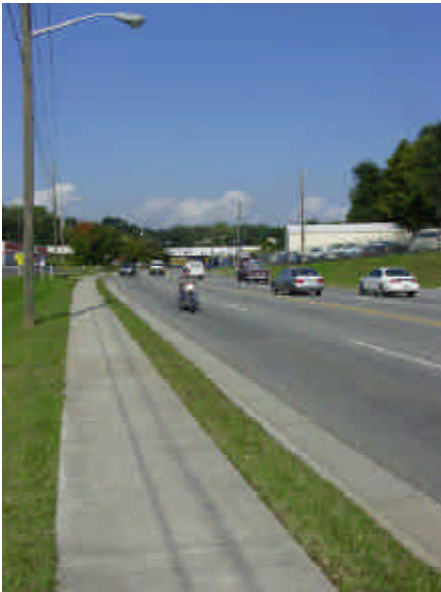
All arterial streets, such as Gus Nicks Boulevard above, should have curb, gutter and sidewalk
