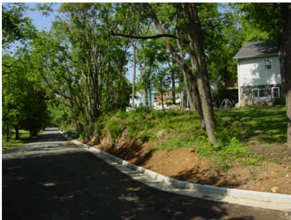
New curb installation in conjunction with new development on Craig Road
