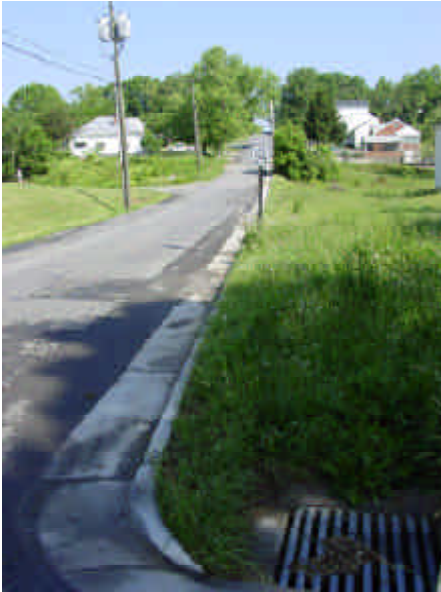
Sidewalk New curb and gutter at 24th Street and Daleton Avenue
