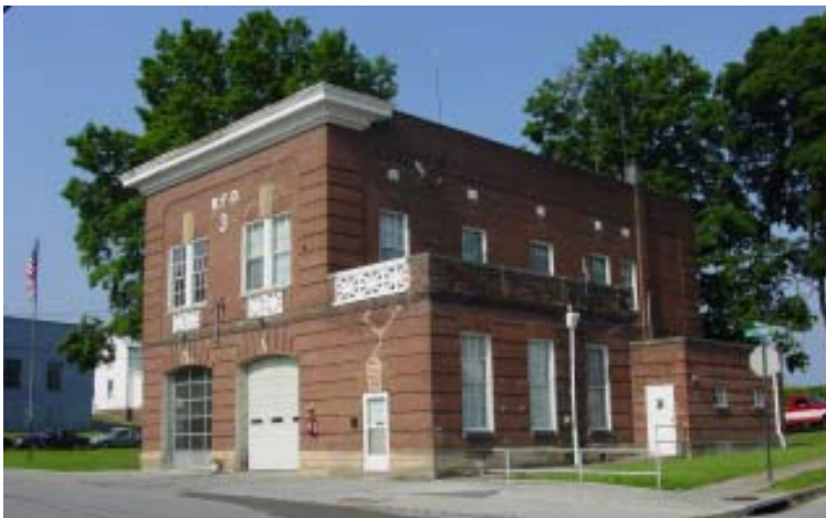
Fire Station Number 3
