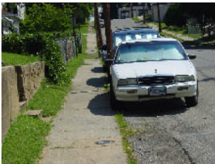
Lack of curb often leads to cars parked on sidewalks which impedes pedestrian traffic.
