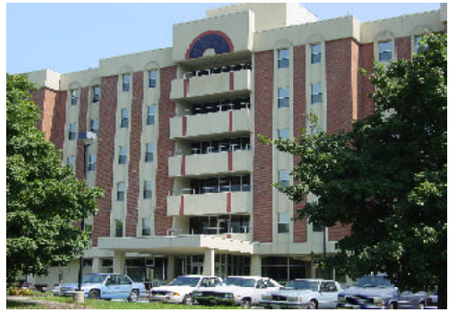
Morningside Manor: located near the village center at the corner of 13th Street and Dale Avenue and in close proximity to two bus lines, it is a convenient location for both residents and their visitors.
