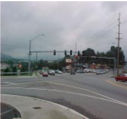
Peters Creek and Cove Road
