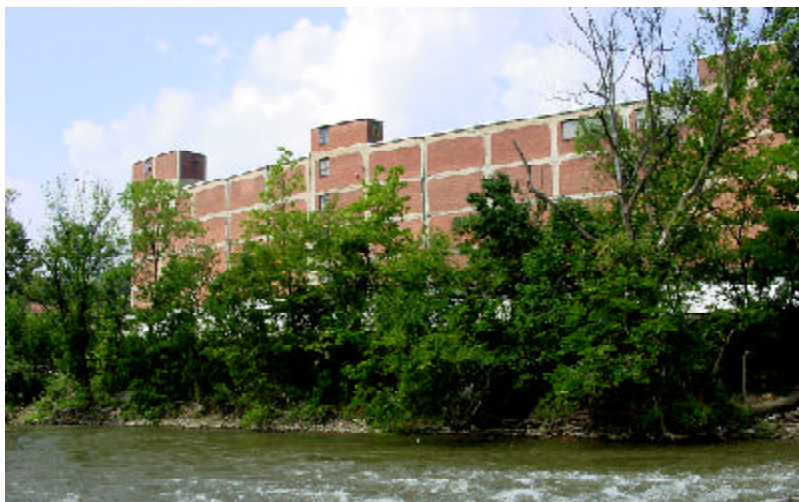
The former ice and cold storage building at the eastern end of Wasena Avenue offers a wide range of redevelopment potential.
