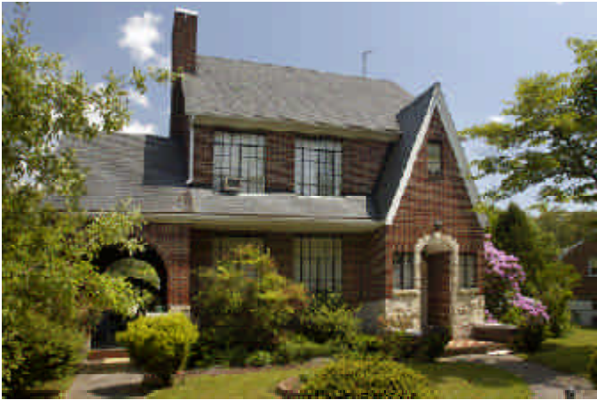
The Tudor Revival style is common in the Williamson Road Area
