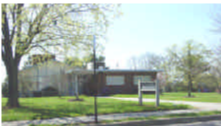
Preston Park Recreation Center
